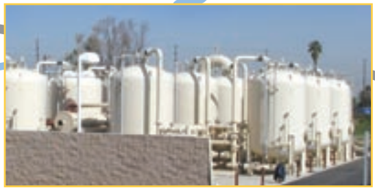
DBCP Treatment Plant
