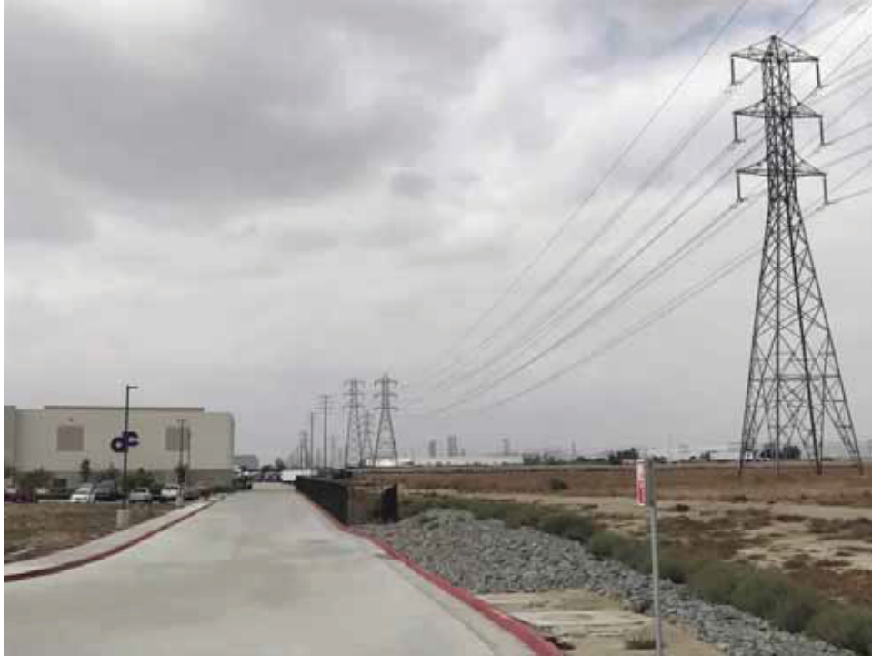
Photo 3: East of Mira Loma Substation.
