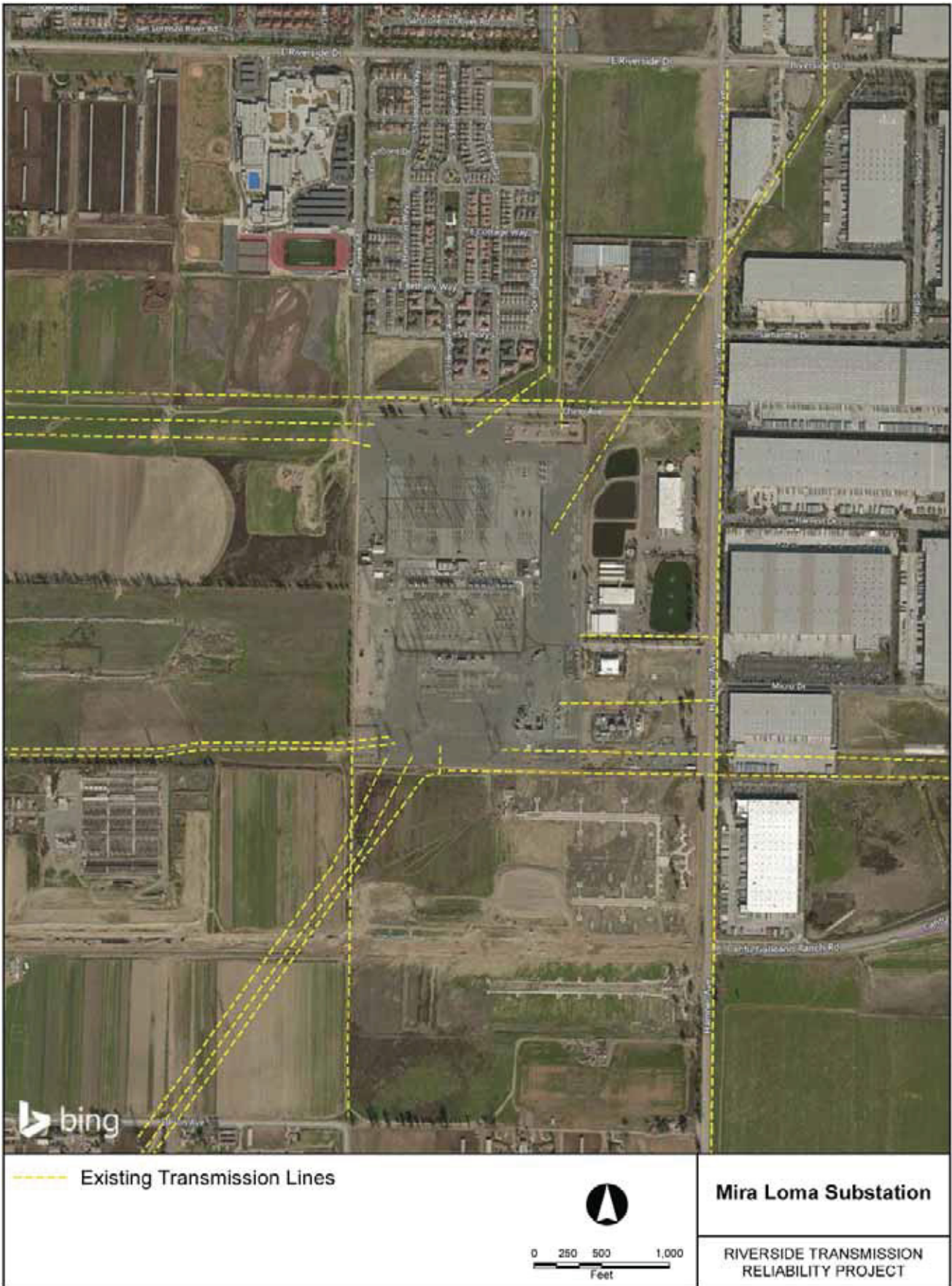
FIGURE 9 MIRA LOMA SUBSTATION AERIAL VIEW
